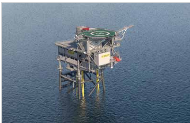
Figure 6. Pilot PosHydon on Neptune Energy's Q13a-A platform [15].
